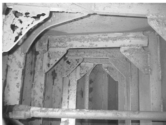
Figure 1: Transverse bulkheads and deckhead
