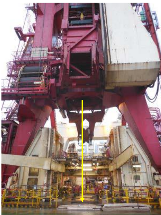
Figure: pipelay tower showing where hammer fell
