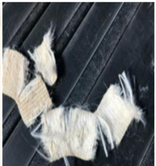
Photo 3 The sling material was found to be fragile and parts easily, suggesting UV degradation.
