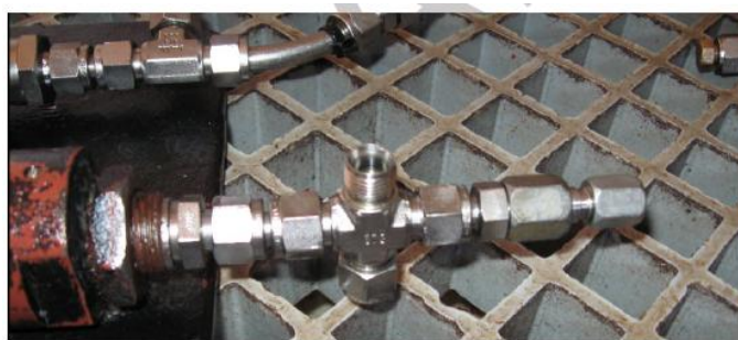
Figure – Open fitting that held the gauge
