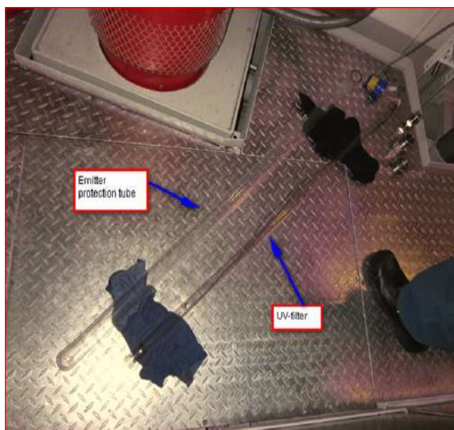
Emitter tube and UV-filter ready to be inserted
