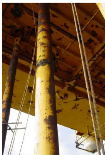
Figure 1 - Area in which rope access hot work was taking place
