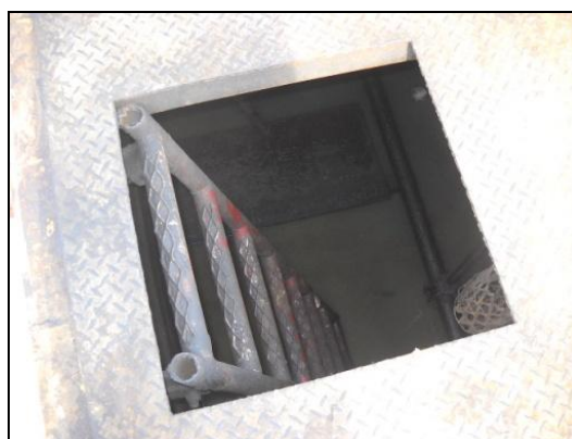
Water tank where incident occurred
