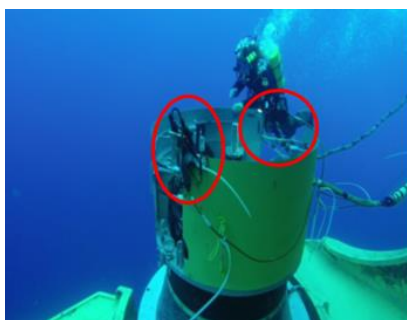
1. Subsea lights fixed to steel support
