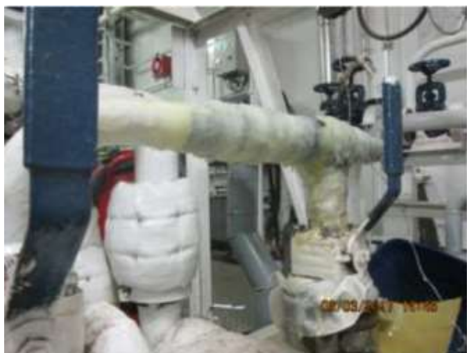
Temporary repairs to the pipe
