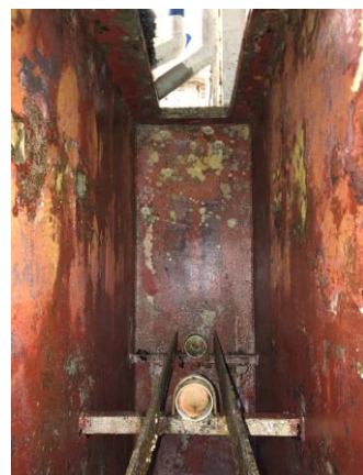
Additional anodes installed
