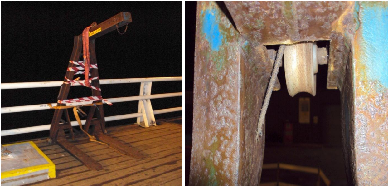
Pallet lifter after parting of wire rope
