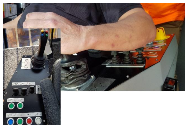
Situation in crane cab
