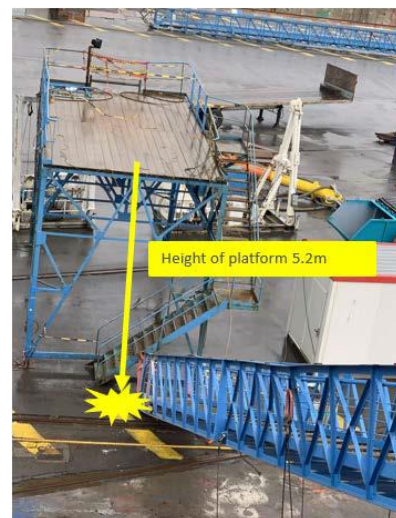
Gangway moves with the vessel and falls off the platform tower
