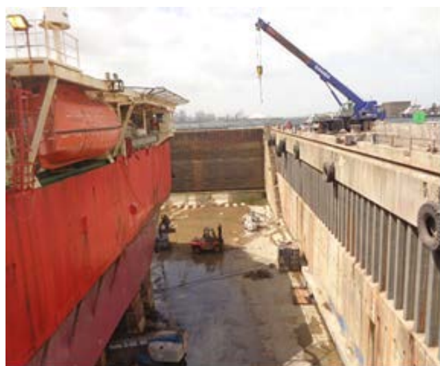
Figure 1: vessel in dry dock with mobile crane
