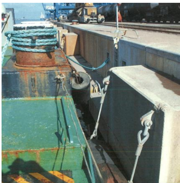
Figure: showing high position of bollard and low position of top hand rail
