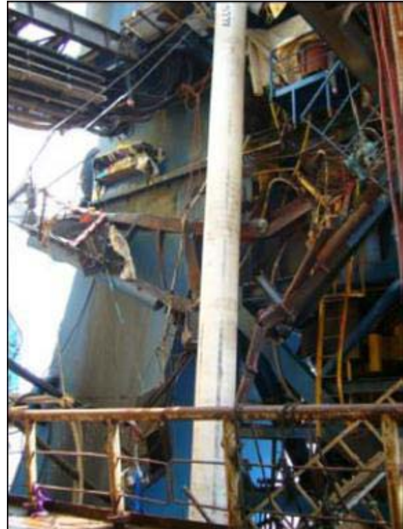
Pipe and wreckage after the fall
