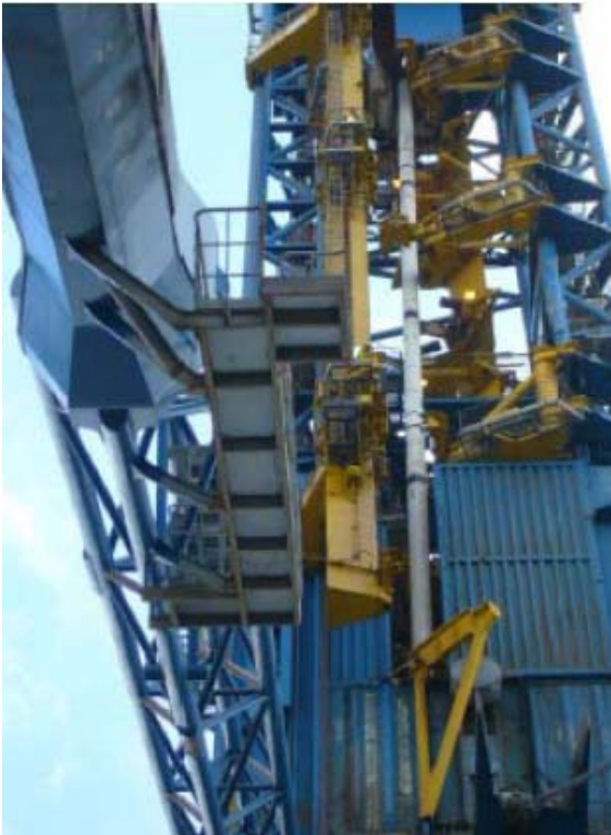
Pipe held in the clamps
