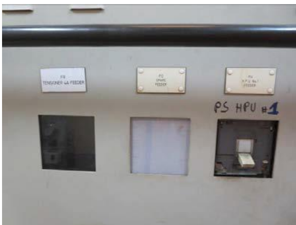
Figure: showing blanks on the switchboard panel where breakers had been removed.
