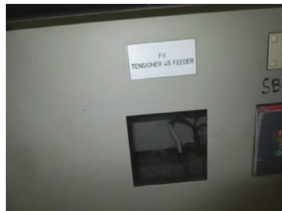
Figure: showing blanks on the switchboard panel where breakers had been removed.
