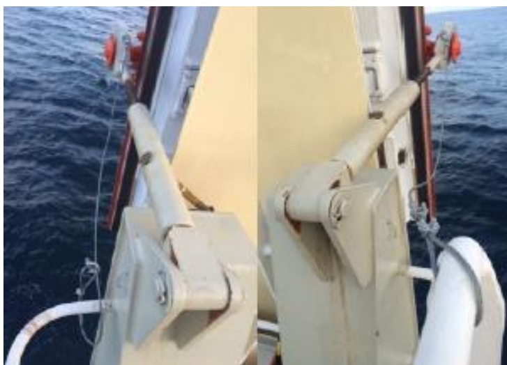
Figure: hooks in use, steel wire secondary securing in place
