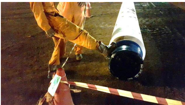
Figure: position of IP when attempting to stop the pipe rolling
