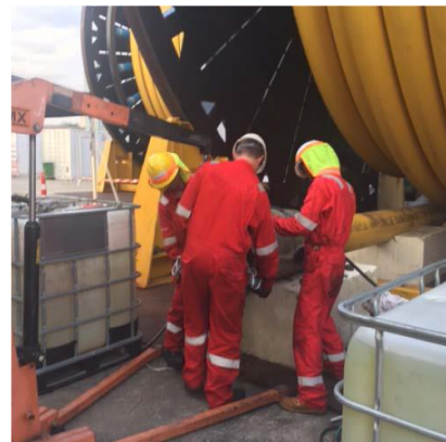
Position of personnel before removal of the 6" pull head.
