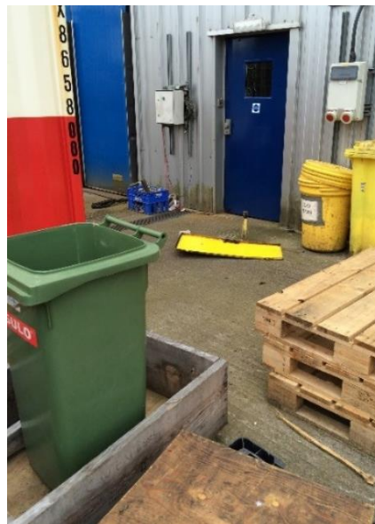
Hood panelling had dropped in front of the main fire exit
