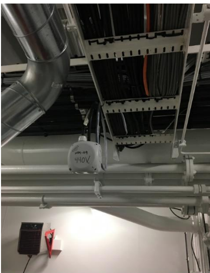
Showing inappropriately labelled live cable
