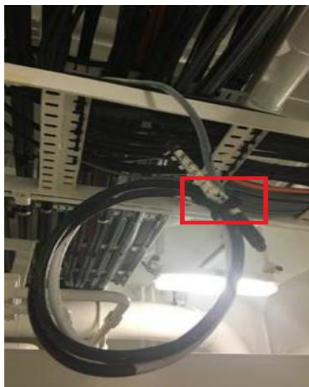
Showing inappropriately labelled live cable
