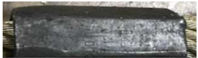
Incorrectly pressed 20mm steel ferrule
