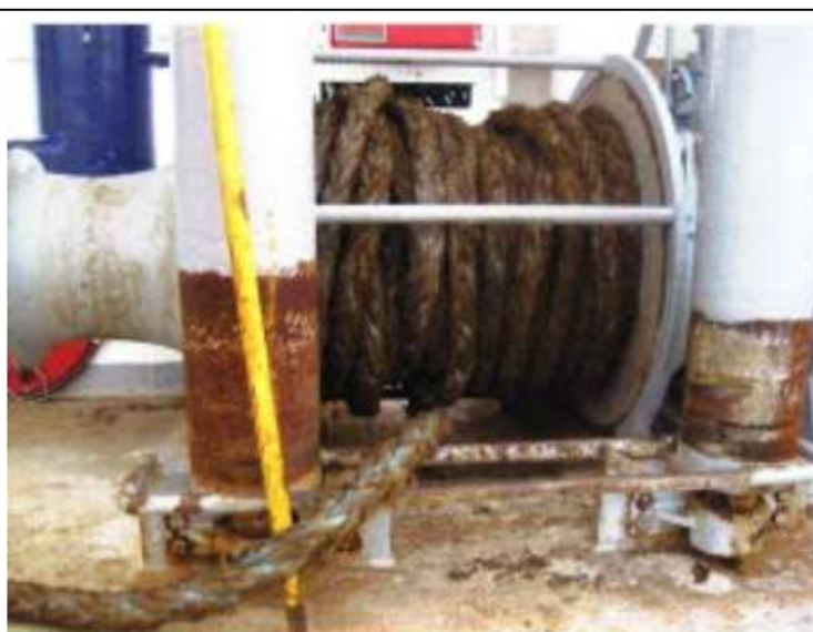
Front view showing mooring line travel to the winch and the crow bar position.
