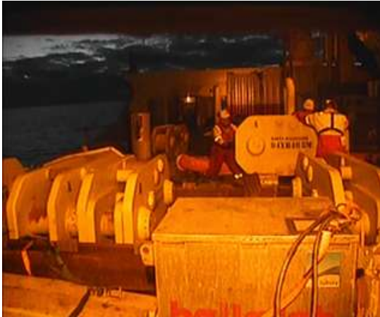
Lowering of H-link into the sled
