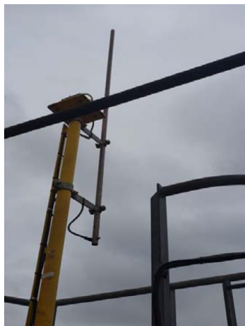
Mast and lightning conductor
