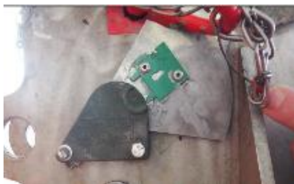
Forward hook after realignment with 'padlock symbol' moved to correctly show safe condition.
