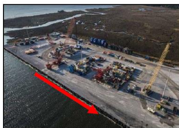
Berthing movement at Core Base
