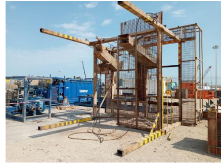
Metal structure proposed for lifting
