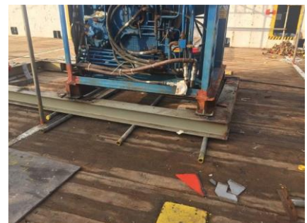
Scaffolding pipes under winch frame
