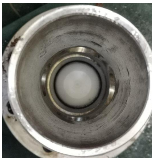
Figure 1 - Endcap Plug detached from float and blocked tank
