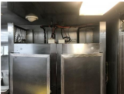
Grate removed showing space above the unit
