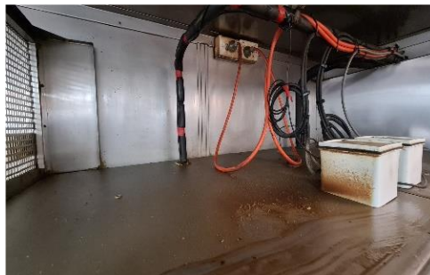
Fat residue on the top surface of the fridge freezer
