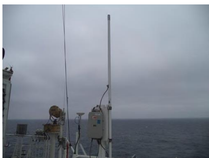
SSB antenna above bridge
