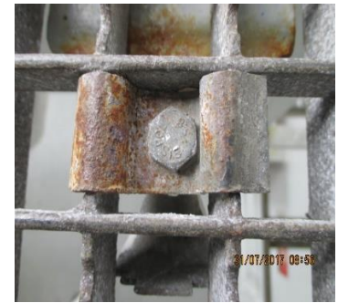
grating clip used for securing
