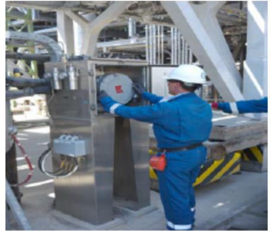
Figure 2: Example of Explosion-Proof Enclosure
