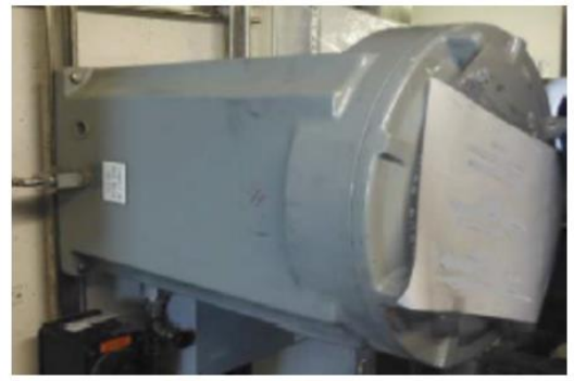
Figure 2: Example of Explosion-Proof Enclosure
