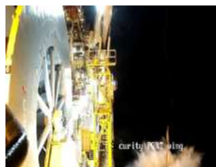
The moment the crane wire parted causing the load to fall to the sea
