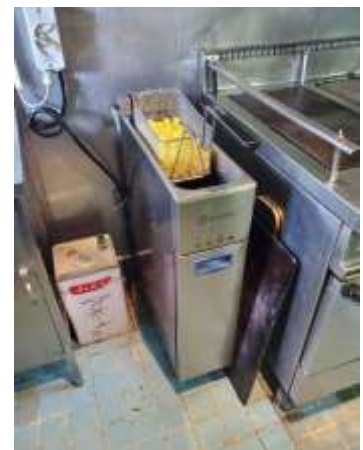
Electrical stove and deep fryer
