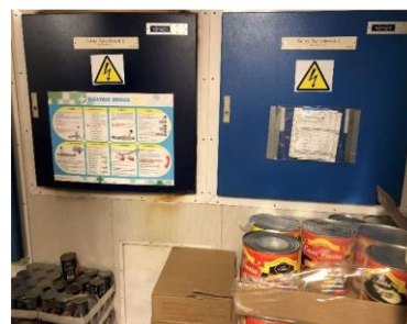
location of the switchboard cabinet where the transformer was installed
