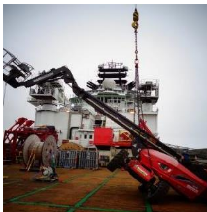
Cherry picker incorrectly rigged
