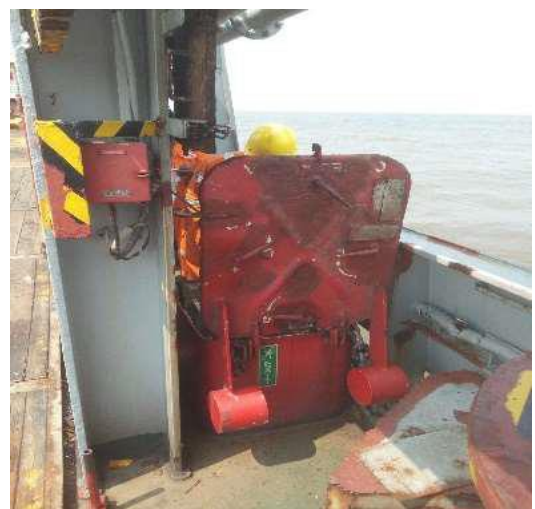
Escape hatch made free after greasing
