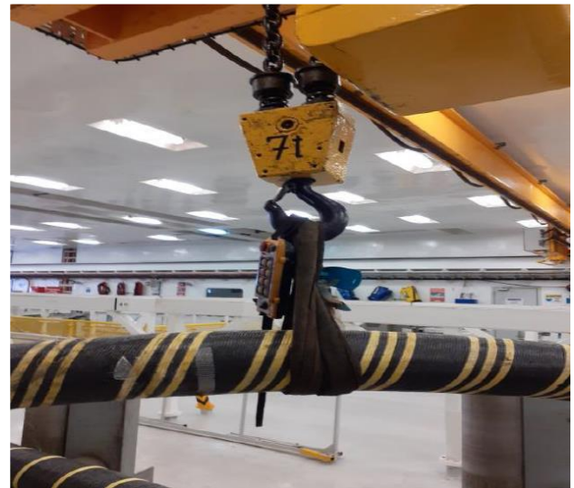
Cable lifted with the deck gantry crane to place the cable back on the roller table
