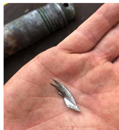
Sheared piece of metal from shackle pin – found close to the winch where the beam was damaged
