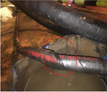
Section of the hose that failed
