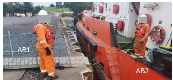
Position of ABs during installation
