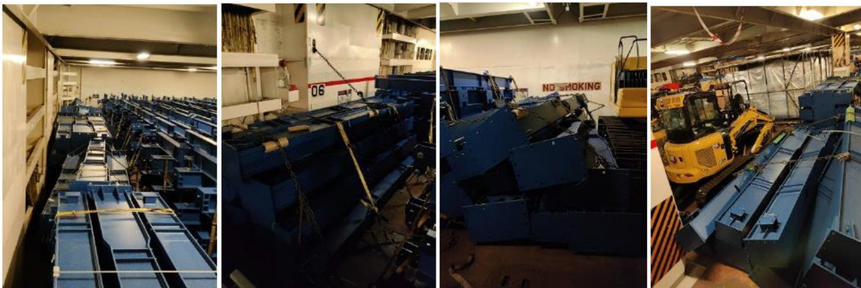
Showing stacks of beams having shifted
