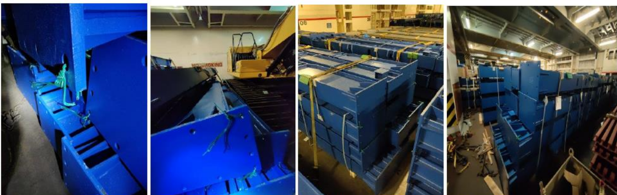
Beams tied with thin metal ties
