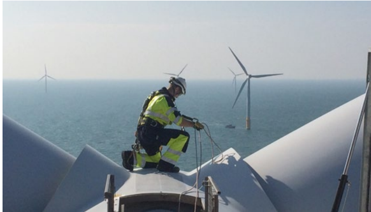
Offshore technician working on wind turbine 300ft above sea level
