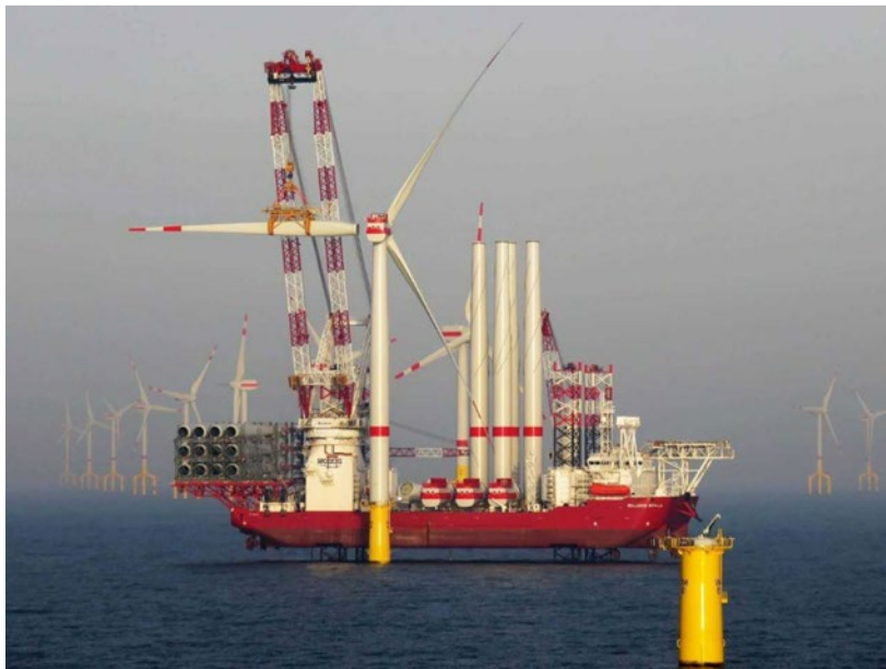
Seajacks “Scylla” installing blades using its 1,500 T crane
