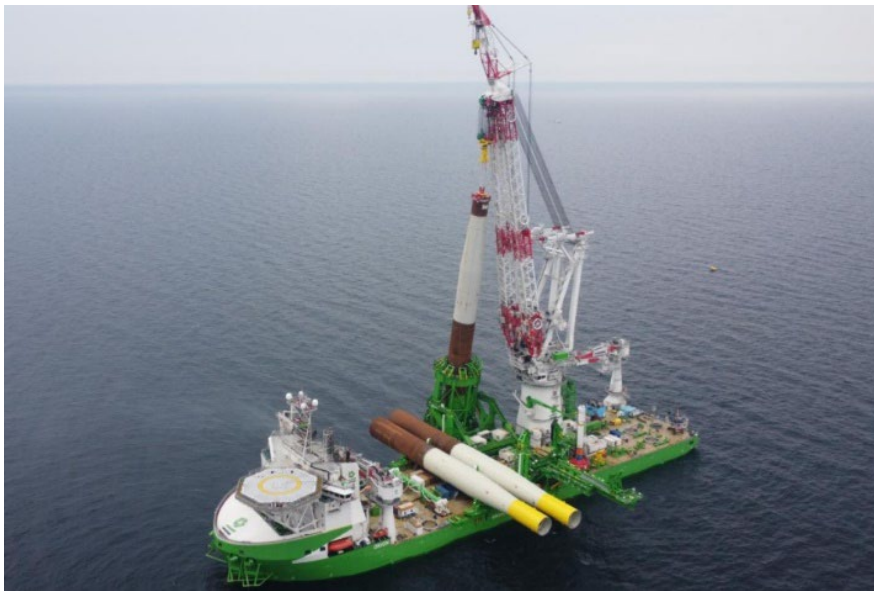
DEMA "Orion" installing 360ft long piles weighing over 2000T with its 5000T crane and tailor-made motion compensated pile handling system
