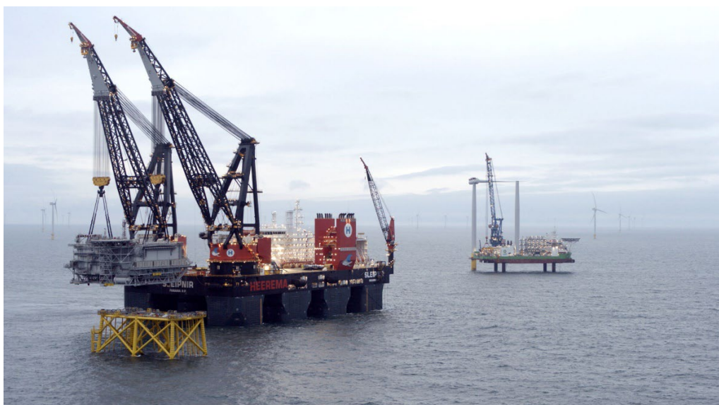
HMC "Sleipner" installing a substation using its twin 10,000T cranes in tandem
