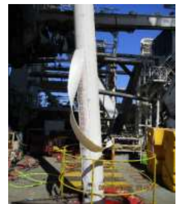
Showing damage to the riser
