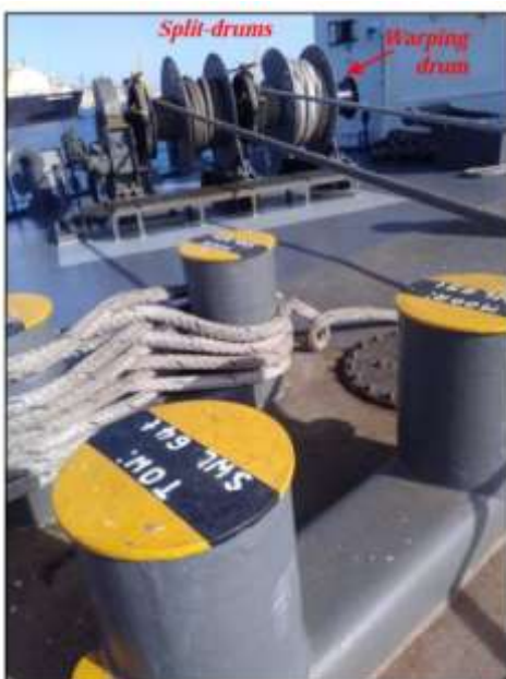
Figure 2: The aft, port side, twin split-drum mooring winch of Mount Everest
