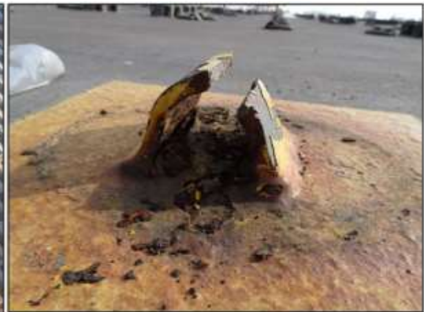
Figure 4. Failed Securing Strap
