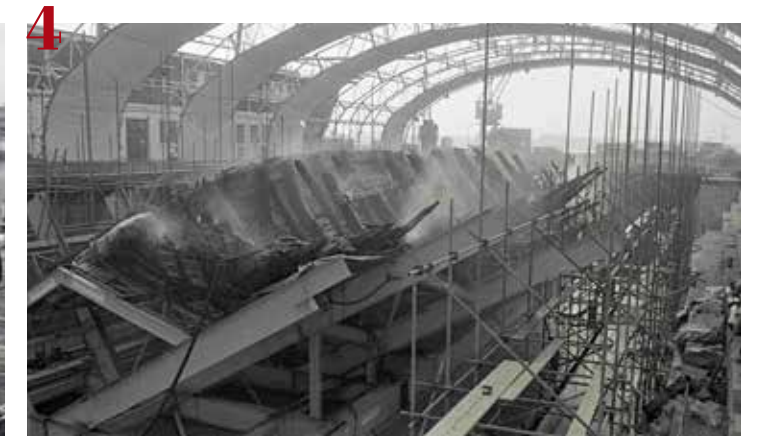
Constructing the Ship Hall over the hull.
