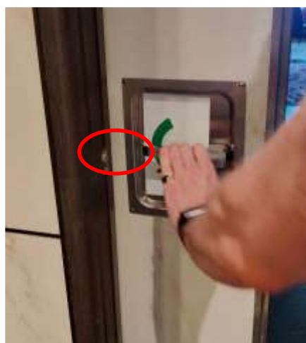
Door operating handle – red circle indicates line of fire
