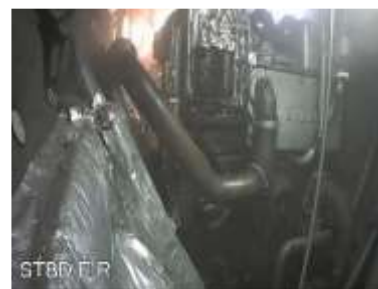
Engine room fire as seen on CCTV
