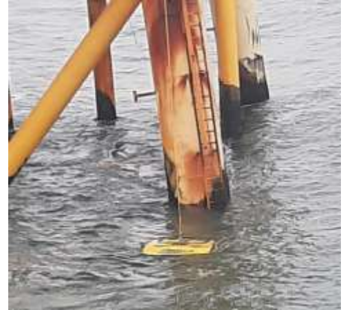
The ROV at the surface just before the tether parted and the ROV drifted away from the platform.
