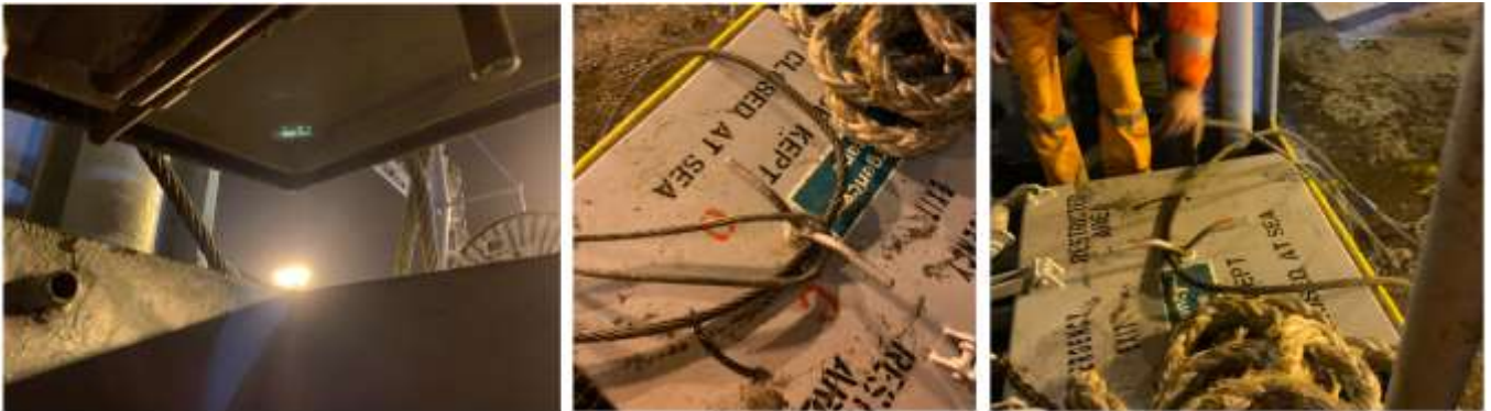
Emergency Exit hatch blocked by wire ropes
