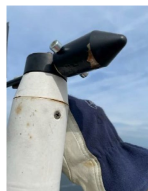
After: new securing method – two grub screws
