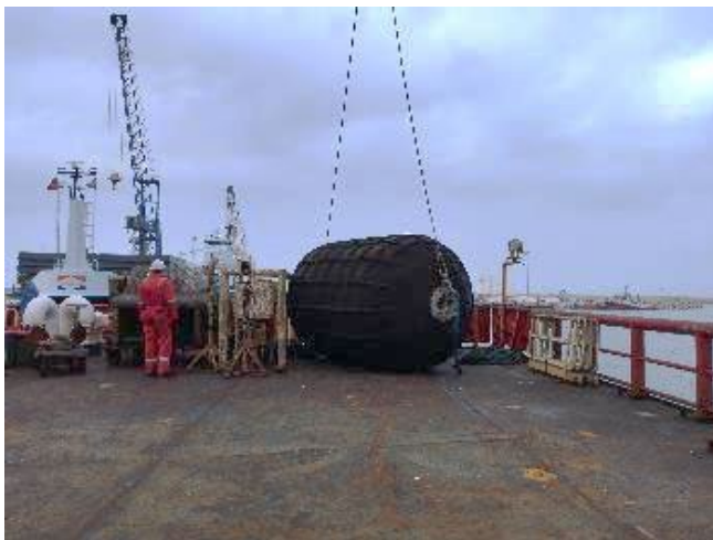
Yokohama fender and bumper bar positioning
