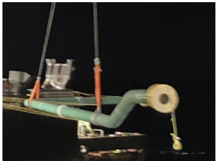
Note the middle leg is not choked, as per the drawing, change not noticed, nor articulated to the divers
