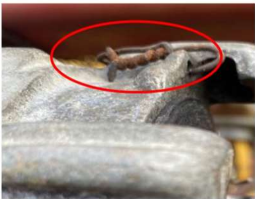
Figure 3 – Baling wire on coupling that released.
