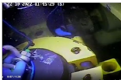
Image 2 – Diver loosening bolts
