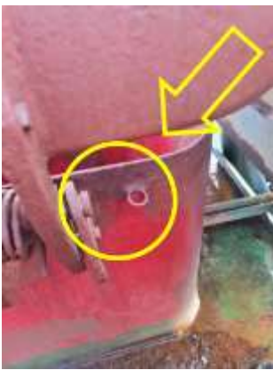
Safety lock pins missing
