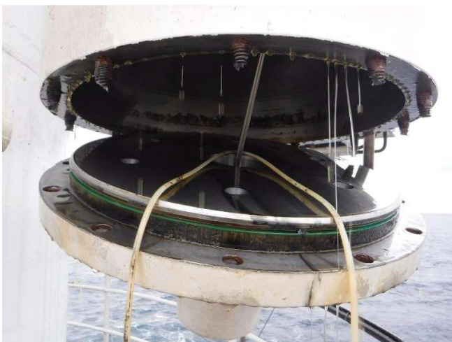
The bottom of the AHC cylinder before the work started on a temporary repair to seal it
